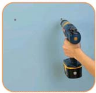
Drill pilot holes at the two marked locations.
