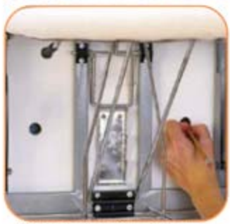
Mark the location of the two pre-drilled holes onto the wall.
