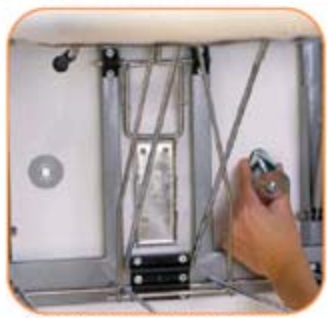
Slide included bolts through cabinet & into wall-tighten.
